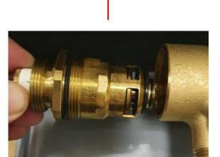
To remove the PICV actuator cartridge, first remove the actuator head by unscrewing the brass nut.
